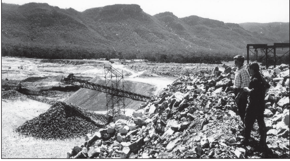
1963: Work continues on the construction of the Lake Bellfield dam wall.
